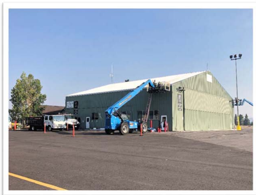
New Roof Installation on Hangar 1 in Summer 2020
