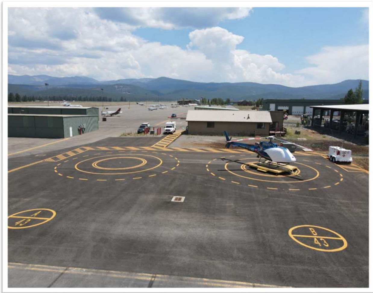
New Emergency Medivac Facility Constructed Summer of 2020.
