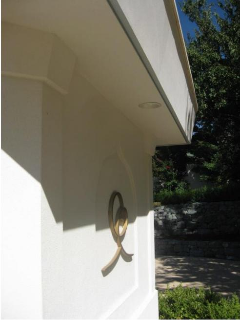
2. Soffit Mounted Down Lighting. No building light-washings or uplighting.
