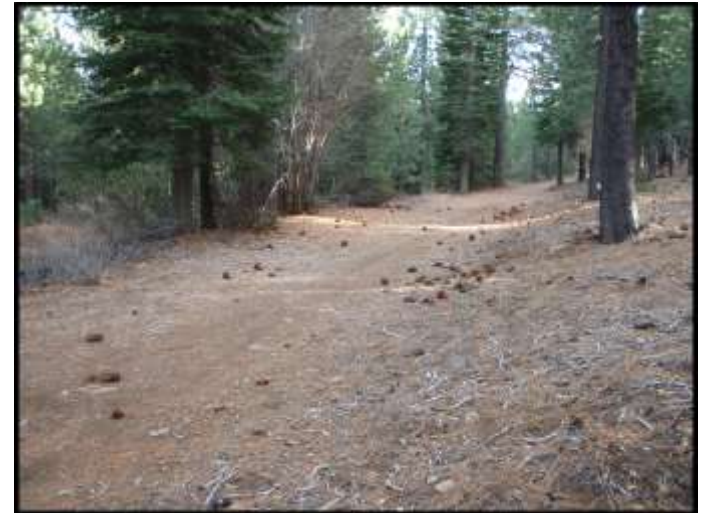
Photo 11d – Typical Road Surface at Lower Project Area near Adventure Center
