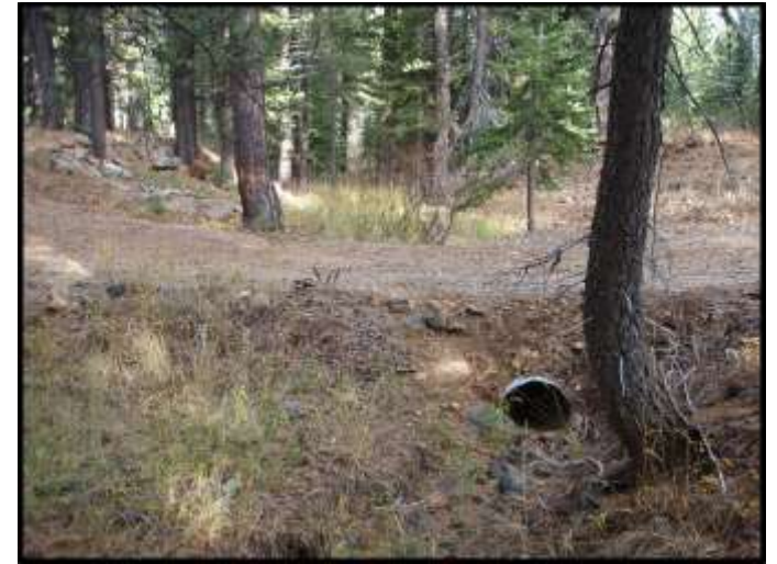
Photo 11a – Existing Culvert Under Project
