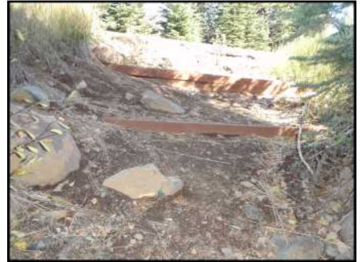
Photo 16c – Start of Spur Trail from Skislope Way (rock steps and rock lined rolling dip) improvement
