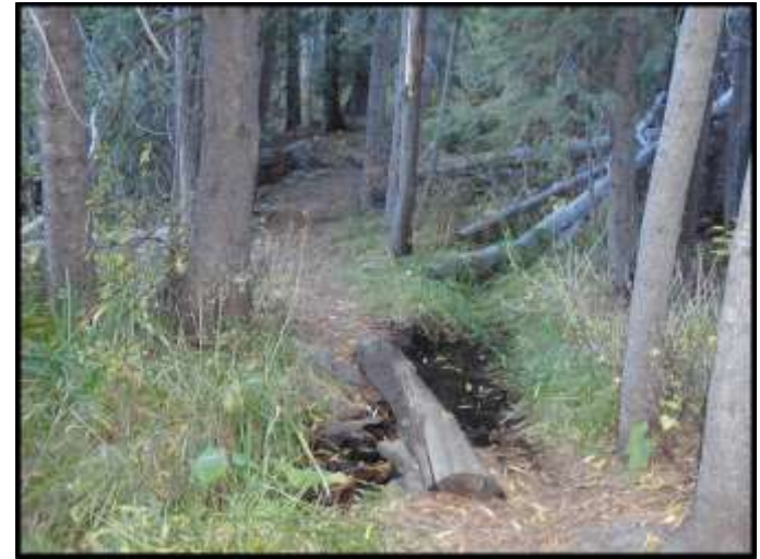
Photo 17c – Puncheons at Existing Drainage Crossings (remove existing)
