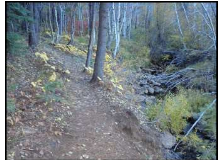
Photo 17d – Decommission Existing Eroding Trail & Realign Uphill from Creek
