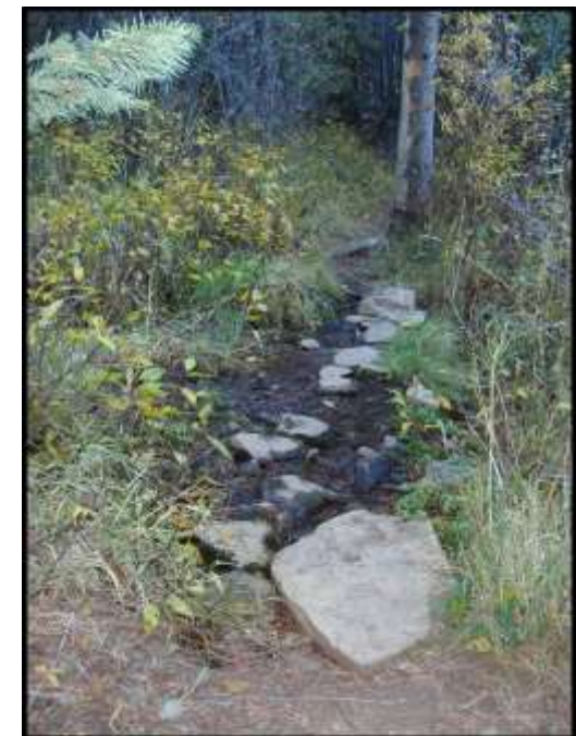
Photo 17b – Punchcons at Existing Drainage Crossings
