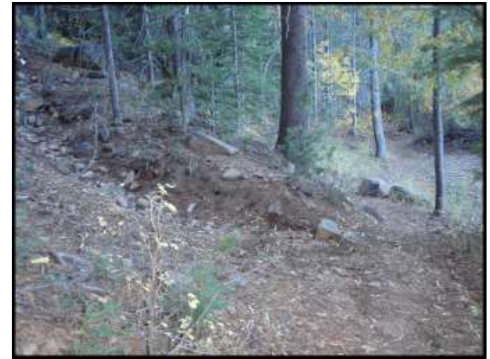
Photo 17a – Location of Rock Lined Rolling Dip at Existing Drainage Crossing
