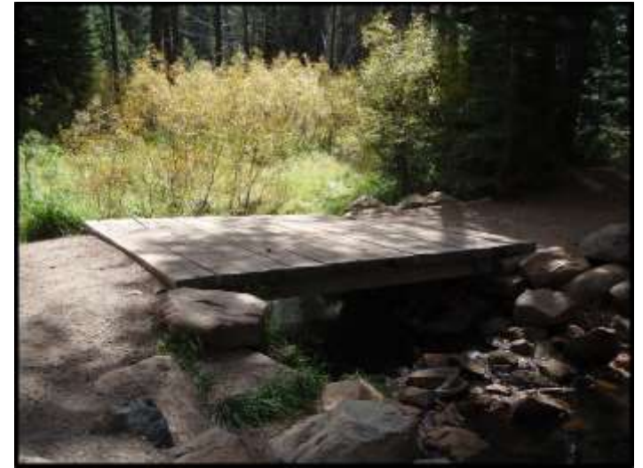
Photo 19a – Bridge Replacement at West End of Project
