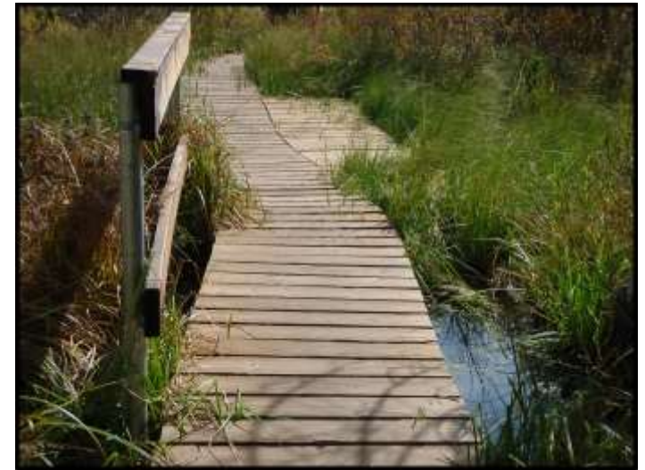
Photo 19c – Boardwalk Replacement at Mid-Section of Project
