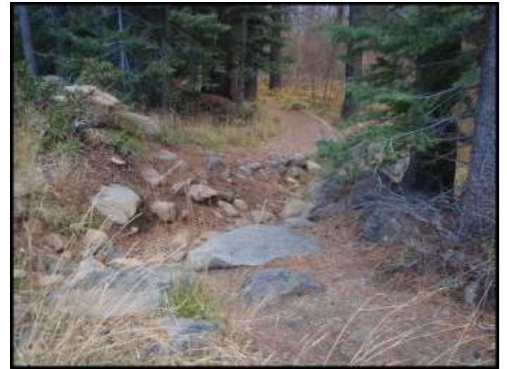
Photo 20a – Armored Swale Near West End of Project
