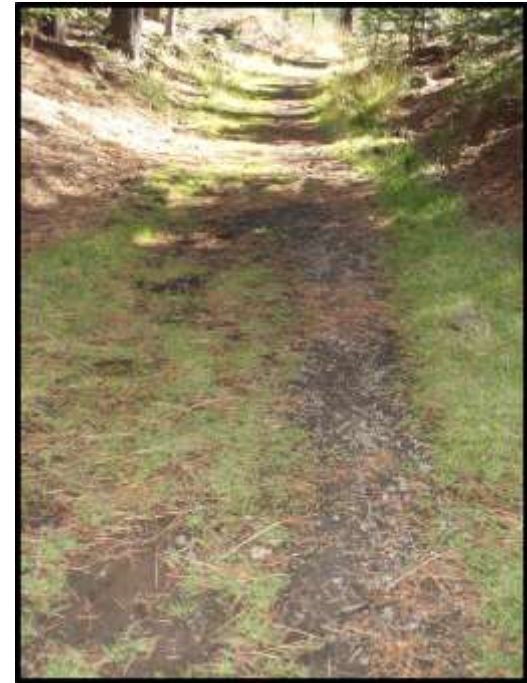
Photo 20c – Turnpike Improvement Mid-Project Adjacent to Northwoods Blvd.
