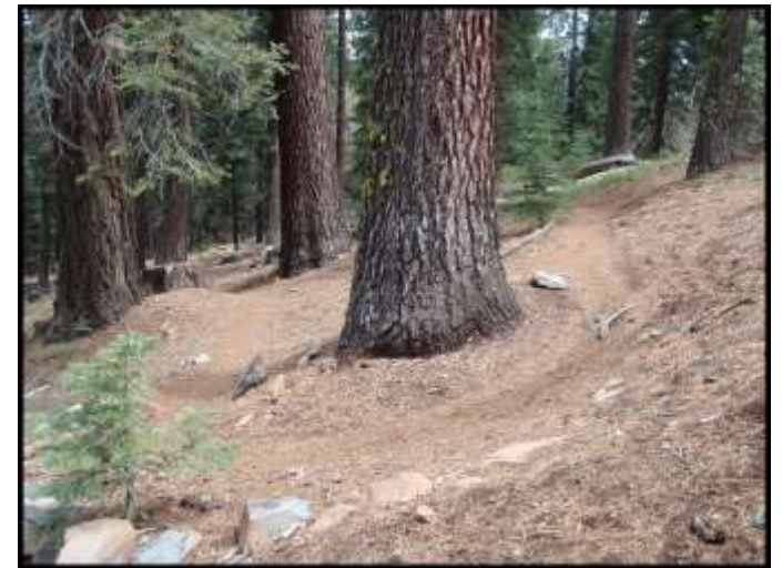
Photo 22b – Trail Realignment & Decommissioning of Switchback of Segment 22B
