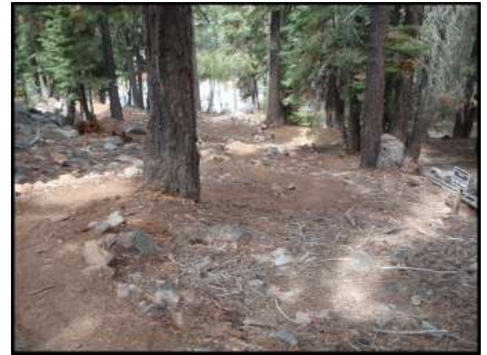
Photo 22c – Looking Down/South of Area of Trail Realignment & Decommissioning of Segment 22C
