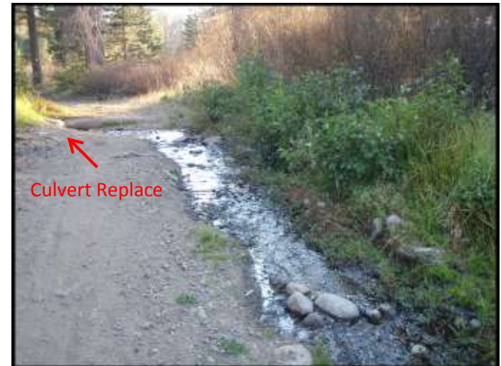
Photo 1b – Culvert Replacement & Roadside Ditch Repair & Improvement
