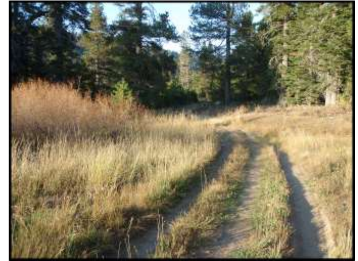
Photo 1a – Rutting Repair Area w/ Drainage Lens at West End of S. Euer Valley Road
