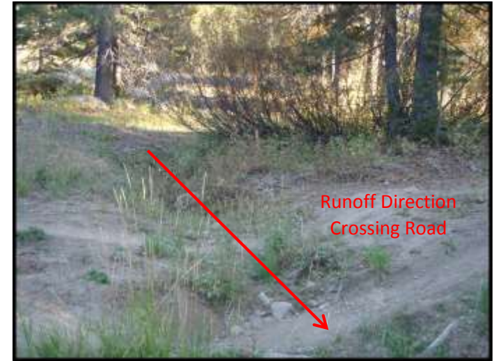
Photo 1c – Typical Condition of Rock Lined Rolling Dip w/ Dissipater Improvement
