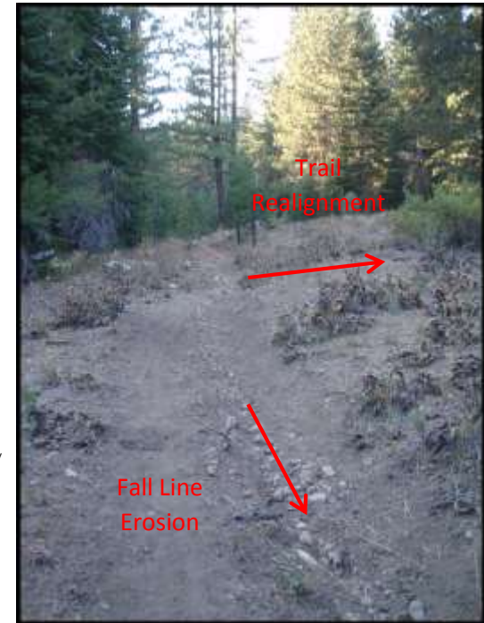
Photo 5a – Fall-Line Erosion at Southerly End of Project Near Intersect w/ Project
